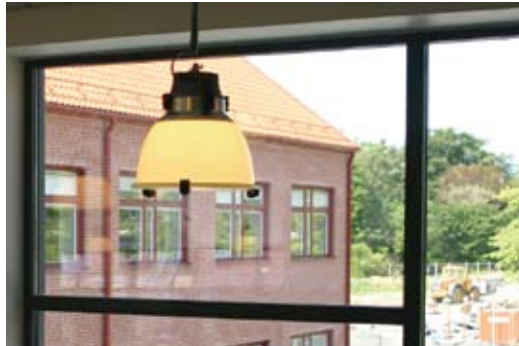
Security system window-contacts are co-utilized by the climate system
